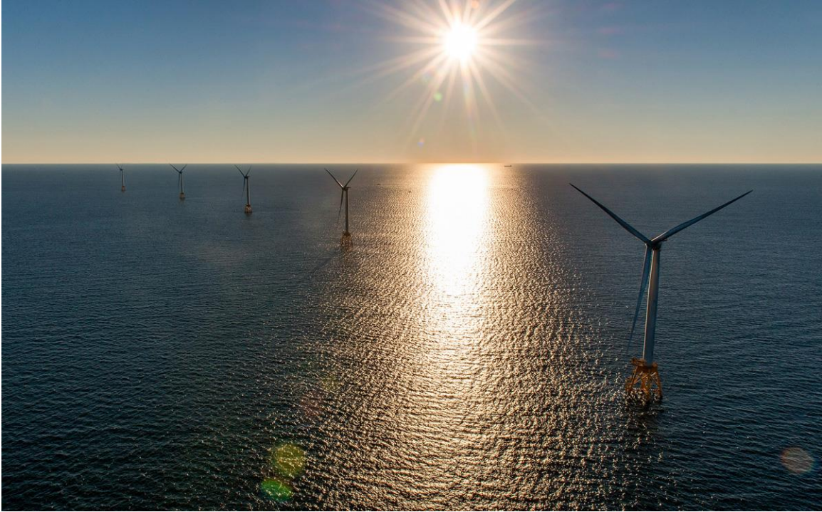
Block Island turbines at sunrise. Source: Deepwater Wind.
